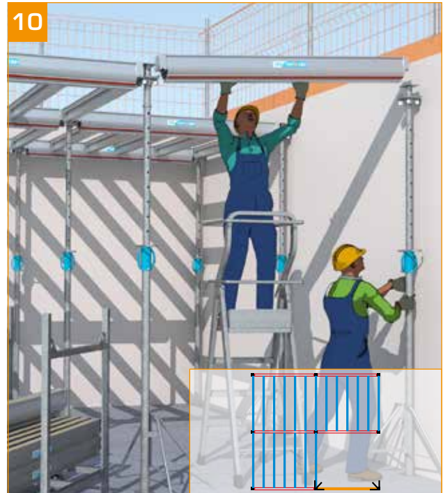
- Set up another primary beam on ST.
