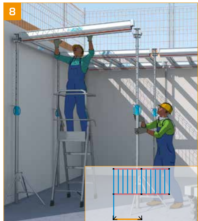
- Set up another primary beam on ST.
