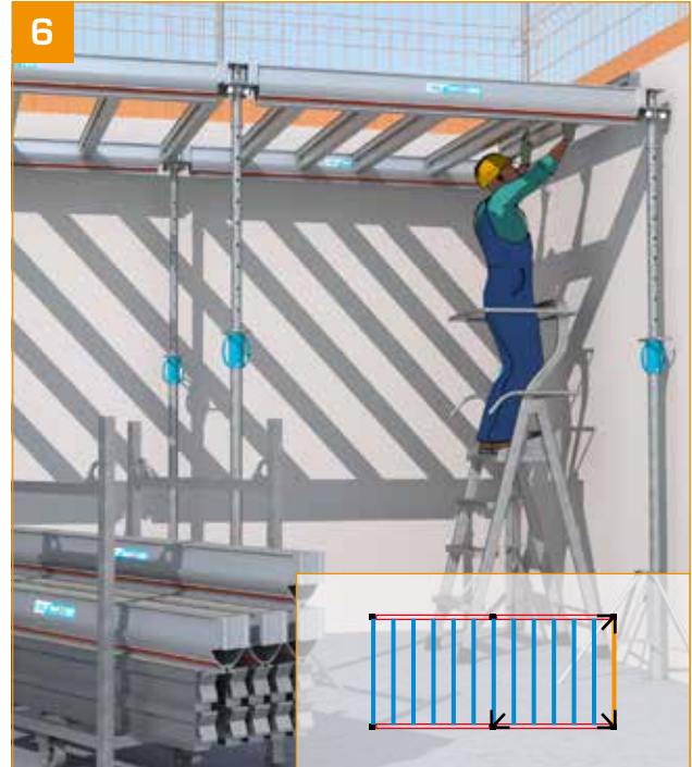
- Finish setting up the secondary beams.
