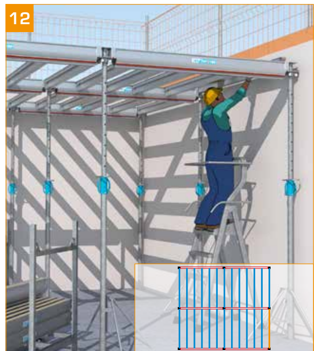
- Finish setting up the secondary beams.
