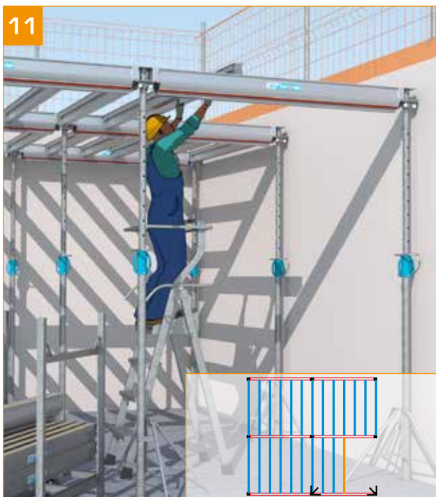
- Move the secondary beams forwards from one to the next, keeping a gap of 39 cm.
